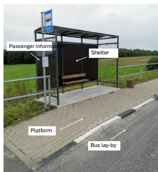
Photo 1. Bus stop with fixtures
